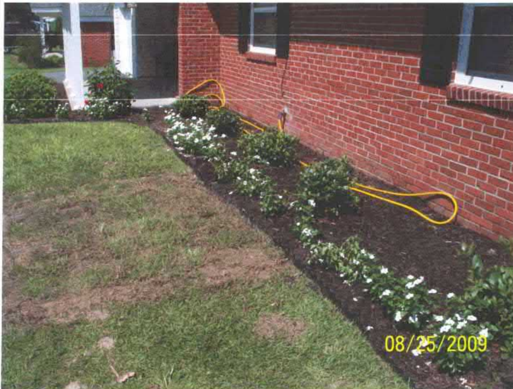
Picture 2: UST 1215Cardinal site after completion of work.
